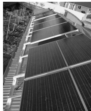
Solar panels (Copyright: Jeff Knowles and DEWHA)
