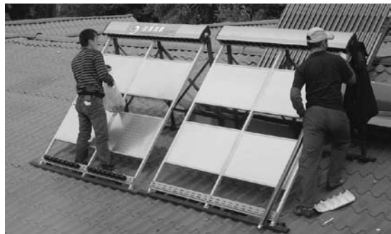
Setting of the solar heating collector (Copyright: A. Nehaenko, PF "EcolDEA")
